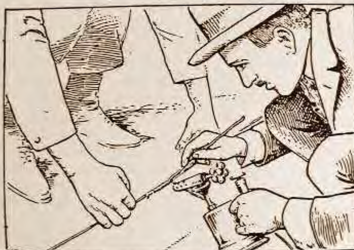
Fig. 117.—Soldering ground wires with torch.
