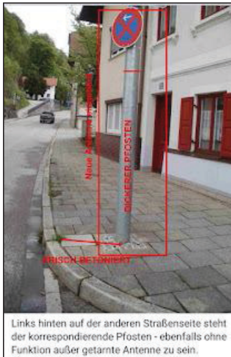
Figure 3: Example of 5G pole in Germany (source: a friend in Germany).
