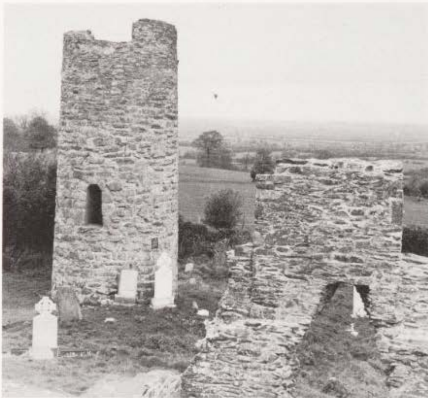
The stump remains of the round tower of Oughterard near Dublin. The round tower originally belonged to a sixth-century monastery founded by St. Brigid. It is made of spalled limestone with a fine granite doorway 2.65 meters above the ground. It is in a graveyard where members of the Guinness family of brewing fame are buried.
